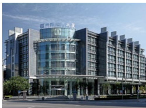
北京 中海地产大厦 China Overseas Property Building, Beijing
